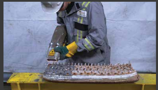
Refractory hanger and boiler tube cleaning
