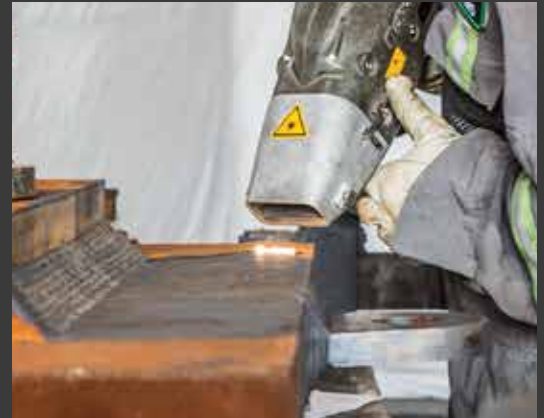
Removal of lead paint
