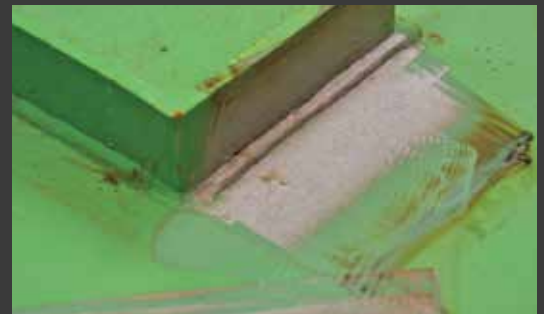
Removal of lead paint
