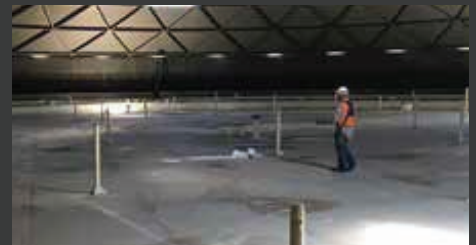
Seal removal and internal floating roof cleaning
