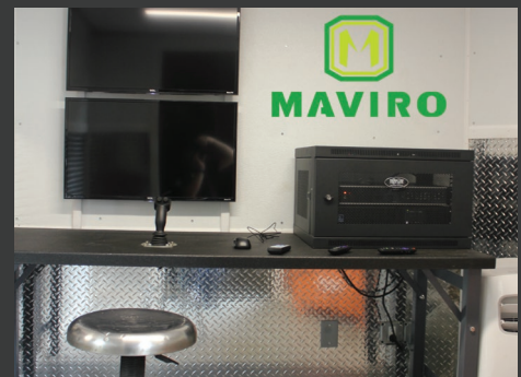
Remotely Monitored Control Room
